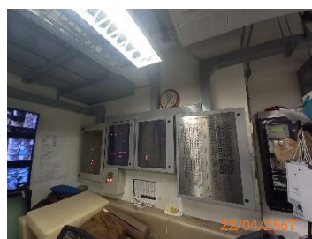
Graphic Annunciator Fire Alarm System
